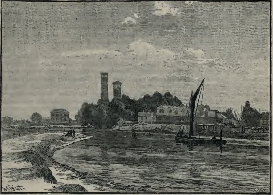
AT LEA BRIDGE.
