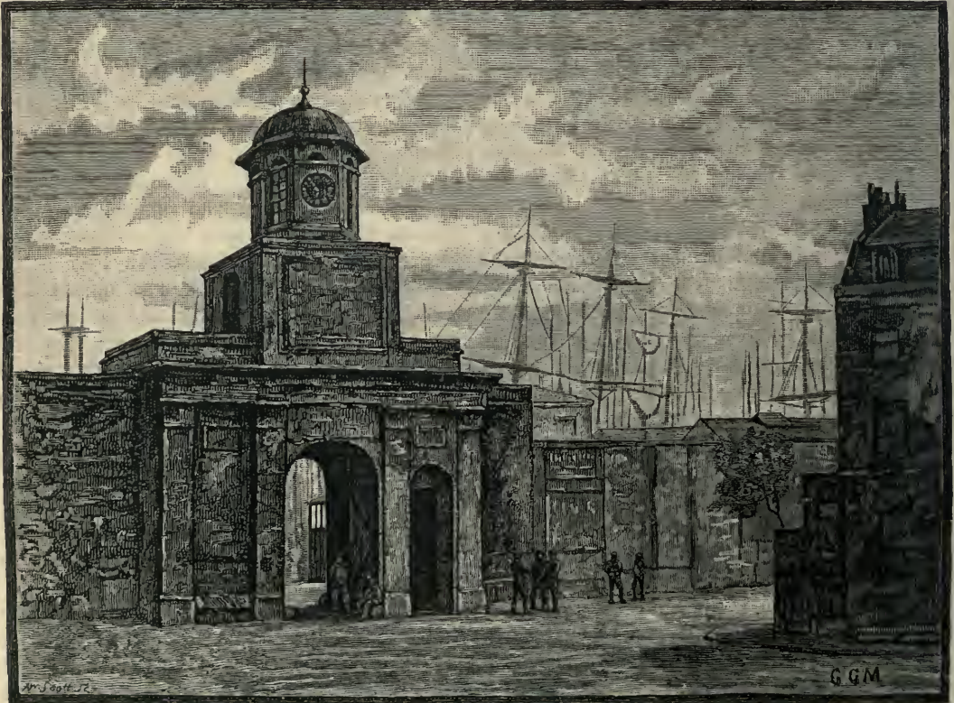
ENTRANCE TO THE EAST INDIA DOCKS.
